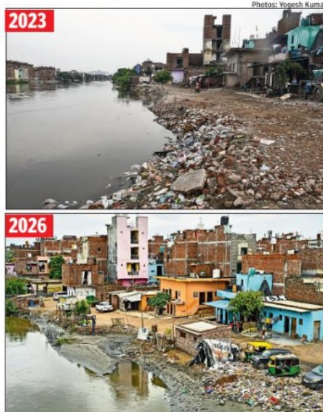
Among the worst-hit by floods in 2023, encroachments have continued to come up along the river's course in Chhajarsi
